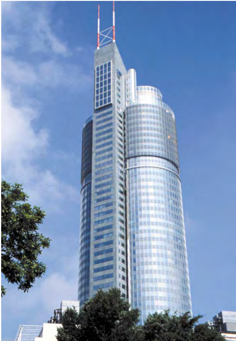
Figure 1: The completed Millennium Tower.
