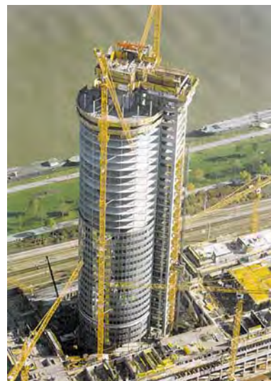
Figure 2: Completing the concrete shell.
