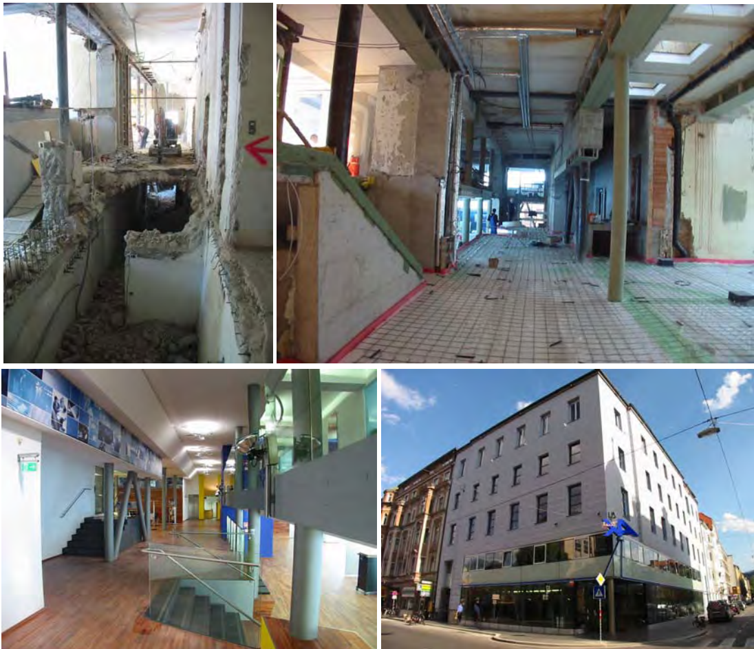
Figure 11. AK office building during and after refurbishment
