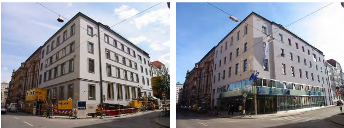
Figure 1. AK office building before and after refurbishment
