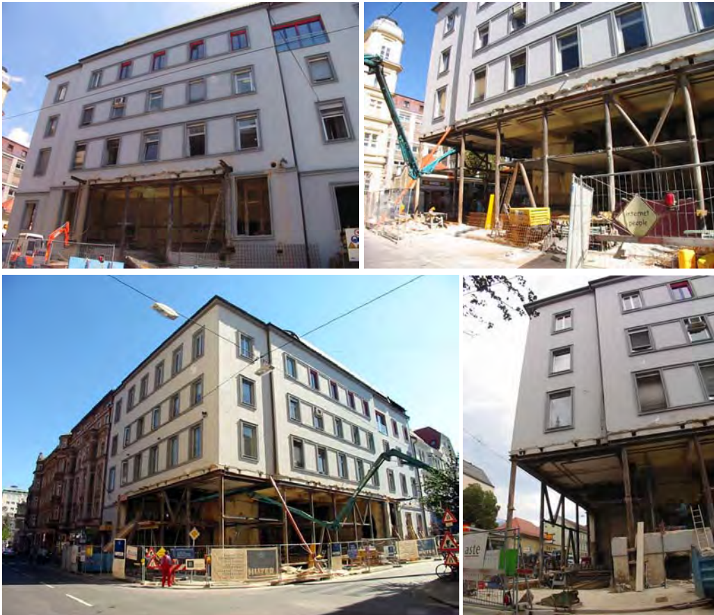
Figure 5. Replacement of external and internal brick walls
